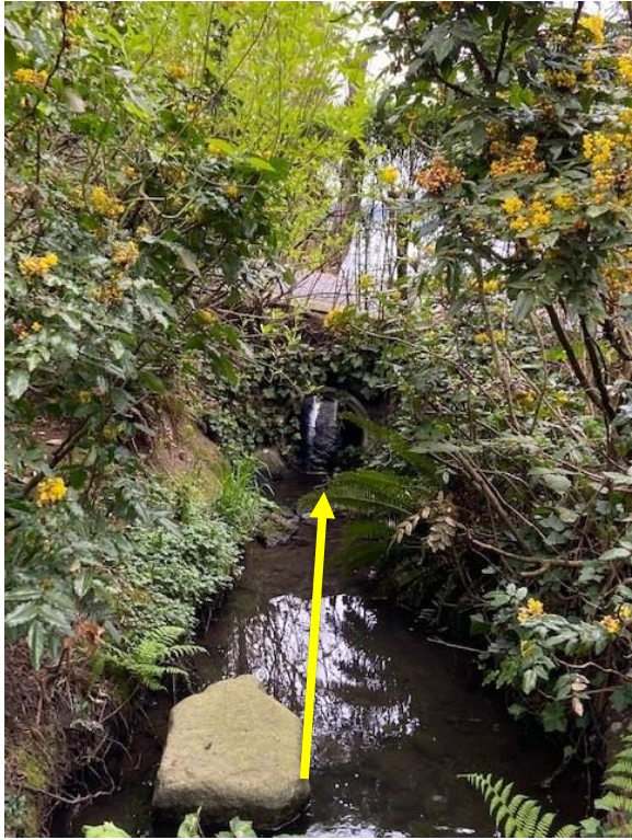
Runoff continues north along 76 th Ave SE through a 24" and 36" culvert.
